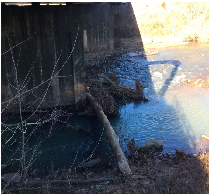
PHOTO 1 Description Drift at Pier 3.
