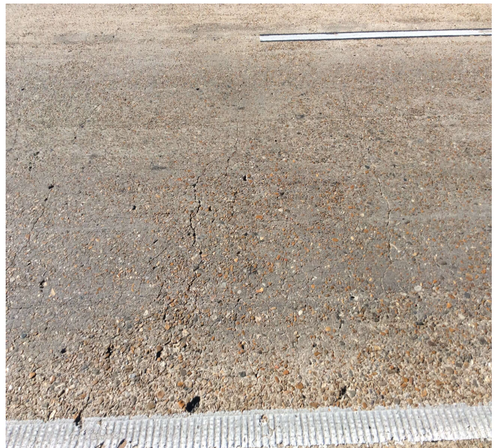
PHOTO 2 Description Typ. Cracking in Deck.
