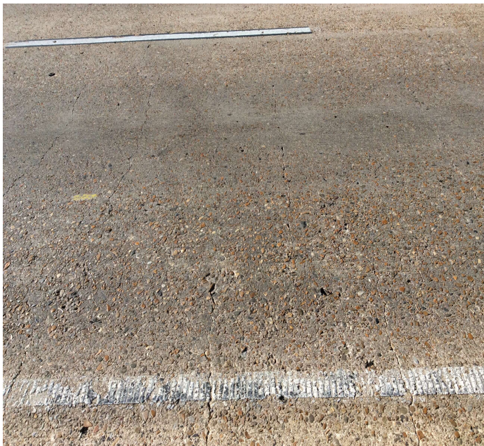
PHOTO 1 Description Typ. Cracking in Deck.
