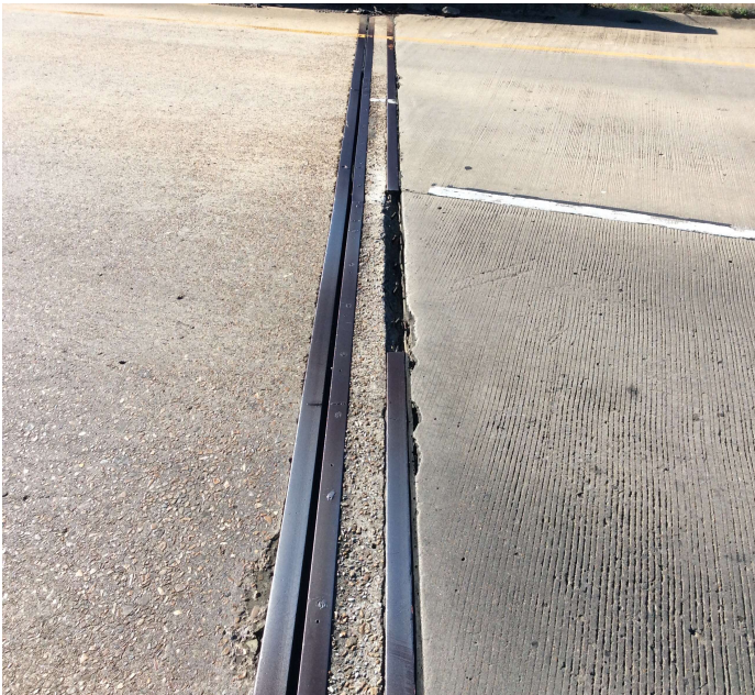
PHOTO 1 Description Joint Armor missing at Abutment 1.
