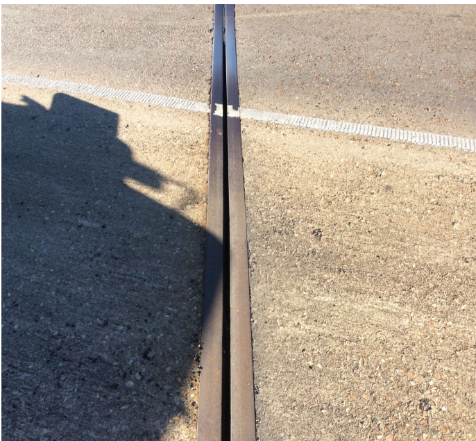
PHOTO 1 Description Joint Seals missing
